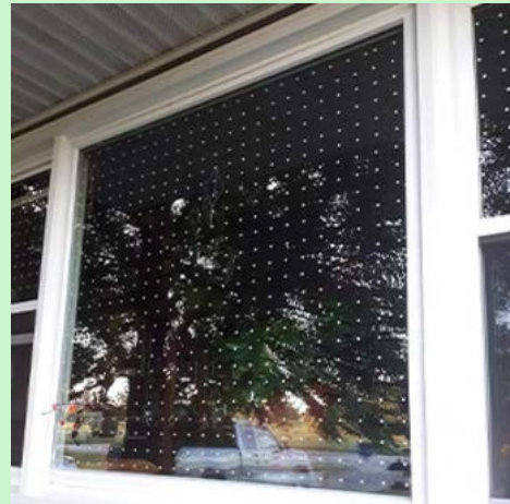
Adhesive white/grey squares installed in strips
