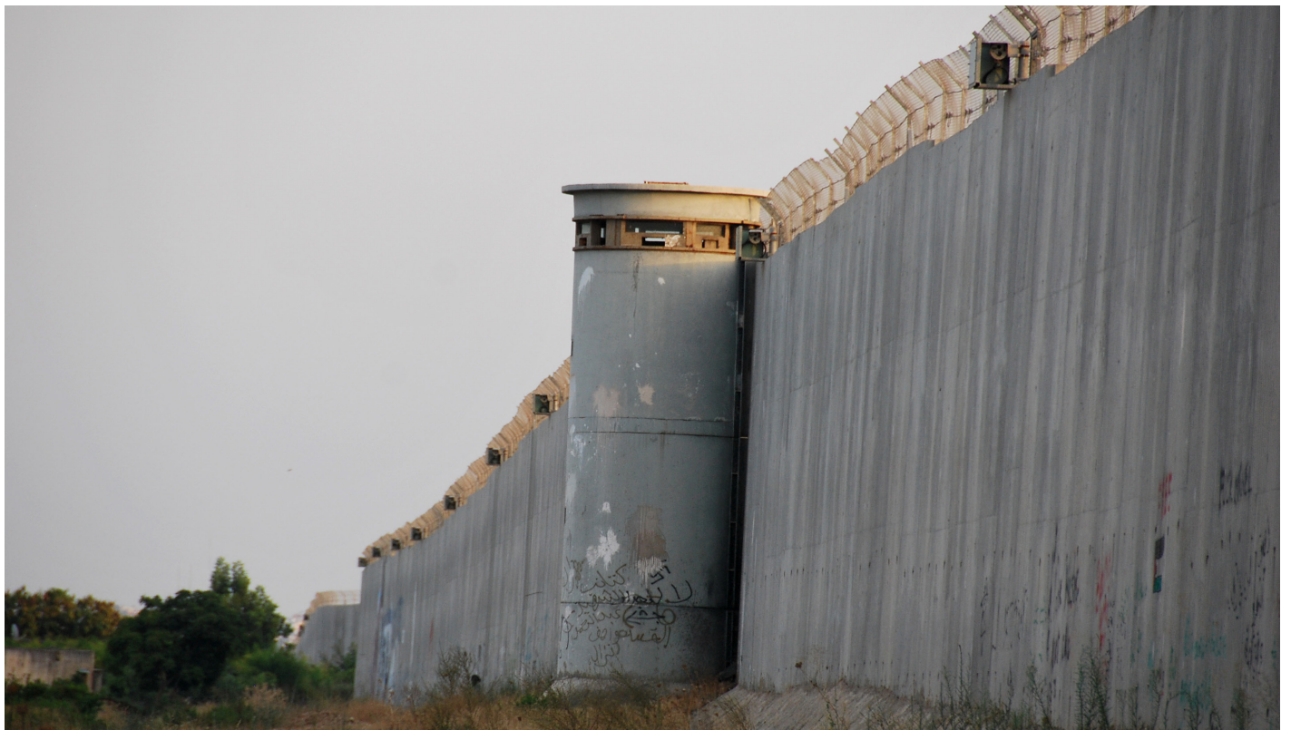
Qalqilyah section of the Separation Wall
